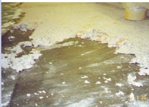
Concrete floor with epoxy coating partially lifted by RemovAll 210
