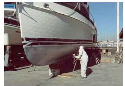
Spraying RemovAll 610 on anti fouling paint on fiberglass
