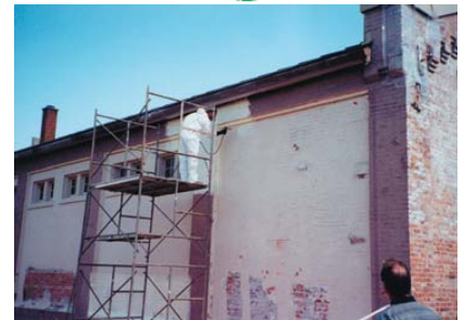
Asbestos based paint being removed from a brick building with RemovAll 310
